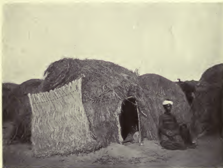
THE FINISHED MANSION. It is put up by two men in a couple of hours, including cutting the grass.
