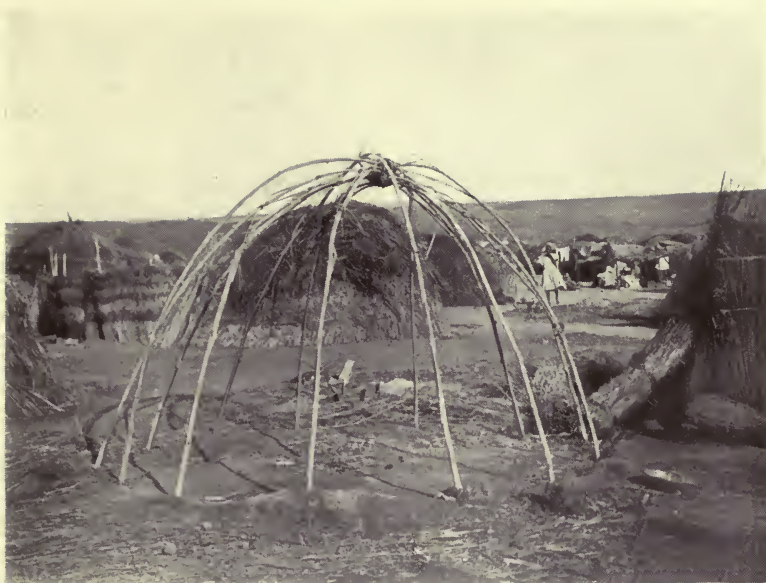
HAUSA HOUSEBUILDING WITH GRASS. The Foundation.
