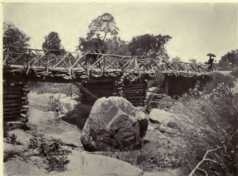
A BRIDGE WHICH IS SWEEPED AWAY BY THE STREAM DURING THE WET SEASON AND REGULARLY REPLACED.
