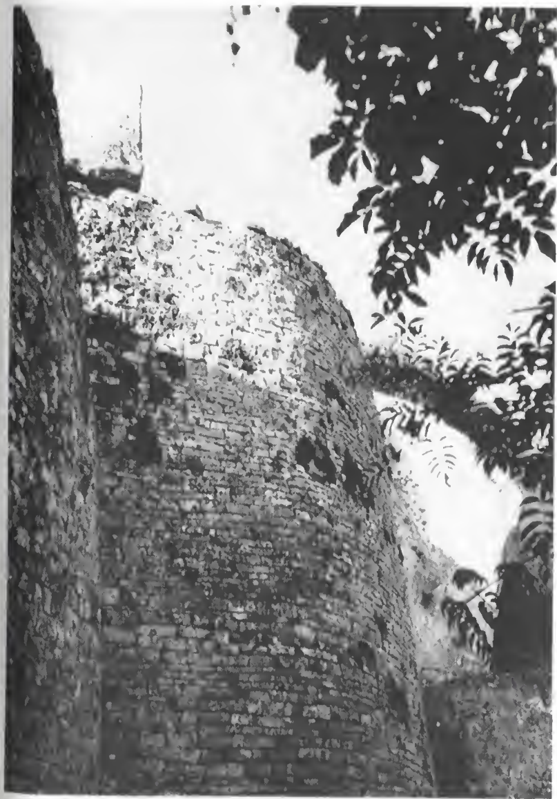
36. Zimbabwe: Cyclopean Architecture. The stones are placed one on the other without cement to hold them together.
